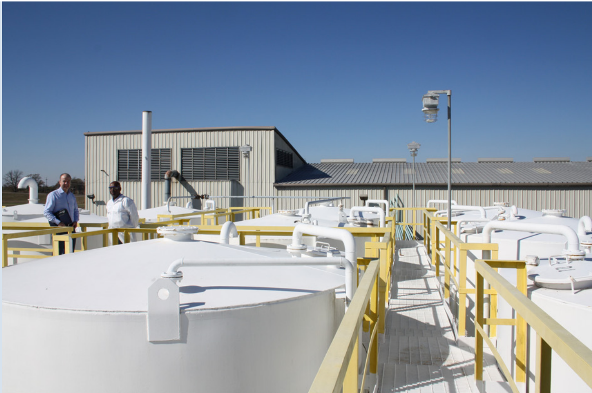
OVERVIEW OF AXEL AMERICAS PRODUCTION FACILITY IN ROSEDALE MISSISSIPPI
