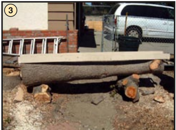
Place the first guide system on the log. This picture shows the Slabbing Rail Brackets, (part number G850) attached to two pre-painted 2 x 4's.
