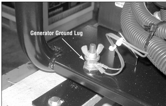
Figure 13 - Grounding the Generator
